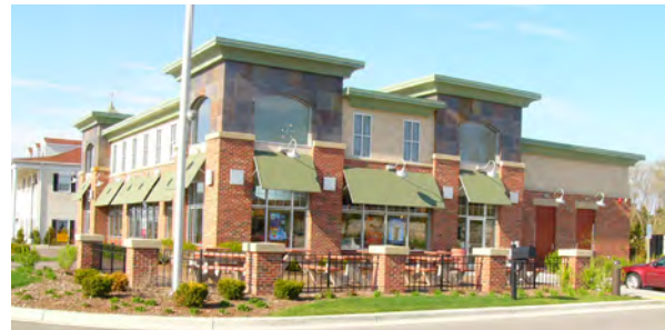
Desired design for a retail building. The color palette includes natural and earth tones. Building uses brick (primary) and EIFS (secondary), and architectural details that breakdown the facade to human scale. There are varying building planes and heights.
