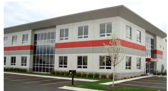
An example of a high quality office building using variations in building color, projections and windows to break up long walls.
