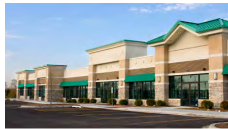
An example of a commercial building using earth tones as the primary color with brighter accent color for awnings and roofing.
