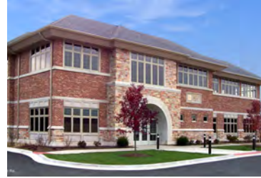
This example shows an office building with a primary facade using brick with stone as an accent material, meeting desired natural color palette.
